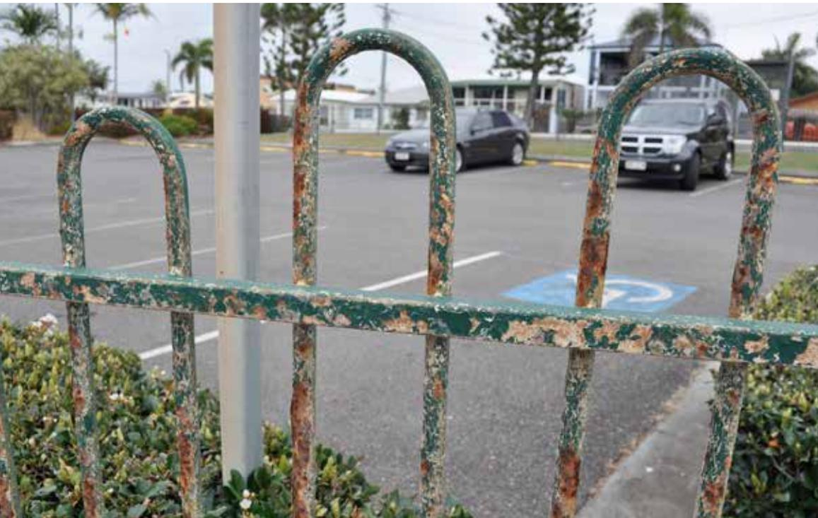
▲ After twenty years the polyester coated fence, across the road from the sea, has also stopped protecting the fence from corrosion. Now the local Brisbane authority will be burdened again by the cost of replacement.
